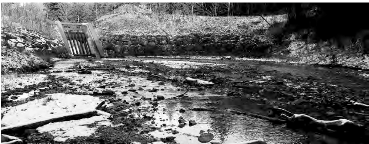
Figure 1.1 – A typical sediment trap with torrential barrier (left) for flow control, with upstream deposition area (Jenbach, Germany). © S. Schwindt.
