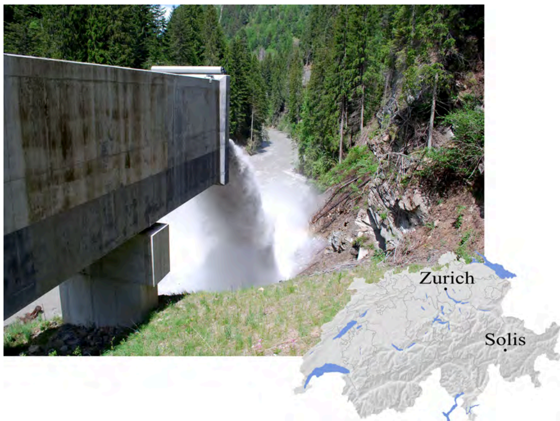
Figure 3.1: Solis SBT during operation (photo by A. Schlumpf, VAW, ETH Zurich) and map of Switzerland to locate it.
