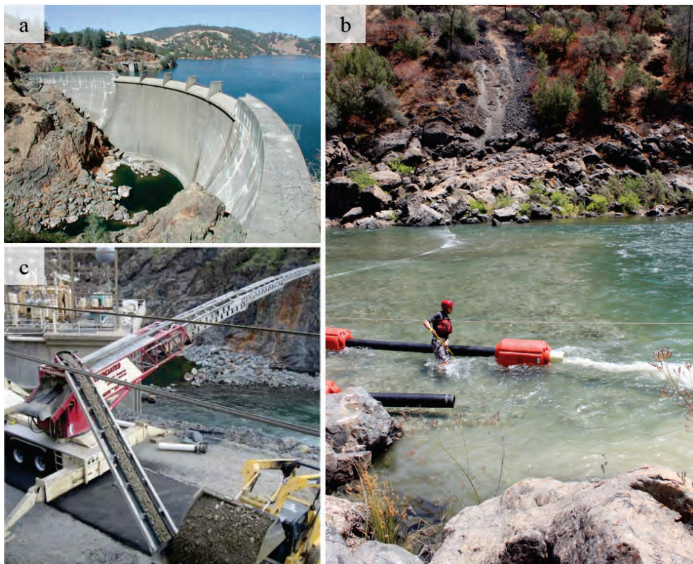
Figure 2.11 – (a) Englebright dam (California, USA), (b) Injection of sediment along the Yuba river (California, USA), (c) material excavation (Pictures by G. B. Pasternack)
