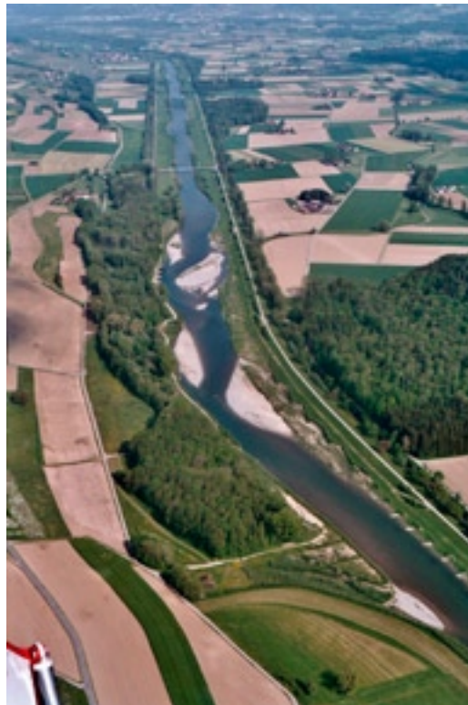
Figure 1.1: Rehabilitated section of the Thur River at Schöffäuli as part of the second regulation of the Thur River (project duration: 1993–2004), TG/ZH, May 2004 (photo: C. Herrmann, BHAtteam, Frauenfeld).
