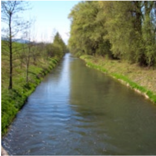
Figure 2.5: Example of a river section poor in structure: the Lichtenstein drainage canal adjacent to the Rhine River at Ruggell, April 2005 (photo: A. Peter, Eawag).
