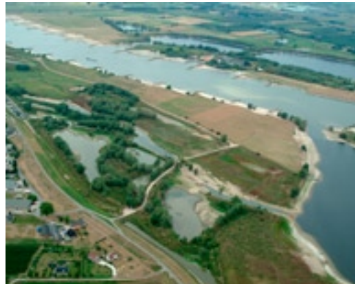
Figure 7.21 (left): Newly created side channel at the Waal River at Opijnen, Netherlands, June 1997 (photo: T. Buijse, RIZA, Netherlands).
