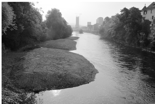
Figure 1. Artificial gravel deposit at the Limmat River in Zurich, Switzerland, view against flow direction (photo by L. Vonwiller, October 2015).
