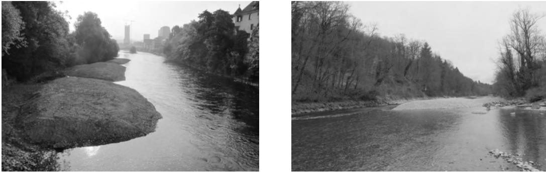
Fig. 1.1.: Artificial gravel deposits at the Limmat River in Zurich, 2015 (left) and at the Aare River in Worblaufen, 2016 (right); Photos: L. Vonwiller
